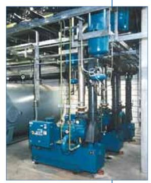
The single-stage compressor types Wittig RO and Wittig RO topline with oil injection cooling supply a constant air flow of high quality virtually without pulsation. In addition to low operating cost, reliability and long life are major features of these types. Due to their long operational life, they have very low life cycle costs.
