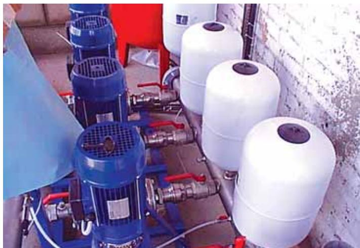
One of the many pressurized pumping stations used with Tecnomatic's systems
