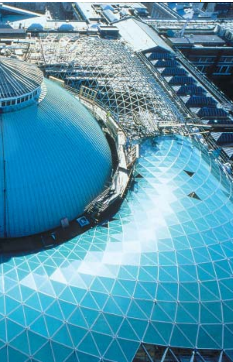
The new roof of the Great Court during construction
