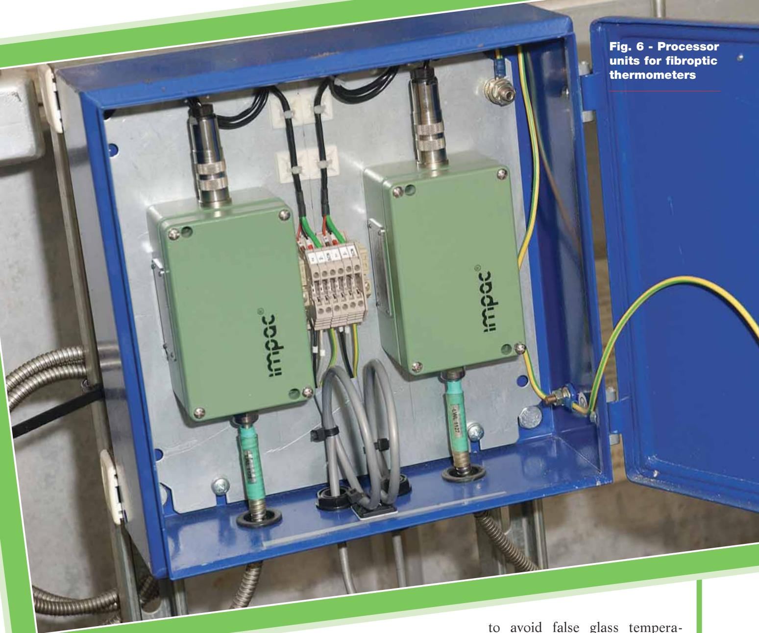
tion is transmitted through the fibre optic light guide to the processor unit. Transmission through the multi-fibre optic light guide is based on the principle of total internal reflection by the boundary surfaces of the glass fibres which is practically free from any losses.
